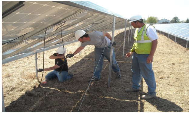
Working on solar racking at the Napoleon solar facility are, from left, Solar Soldier's Joshua McFadden of Johnstown, Ohio, and Justin Harris of Columbus, Ohio. They're working under the direction of Eric Wiemken, site lead for AP Alternatives.
